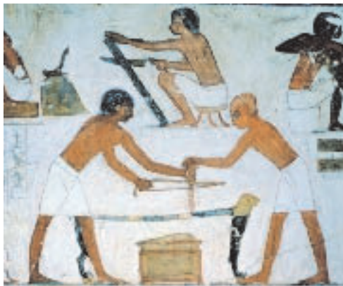
Carpenters at work, from a painting in an official's tomb
